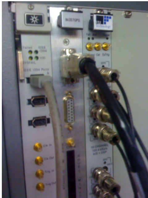
Figure 2.5 - Close view of the three boards. In the middle, on the BC537gps, we can see the 15-pin connector (still free). Above we have the connector and cable of the GPS antenna.
